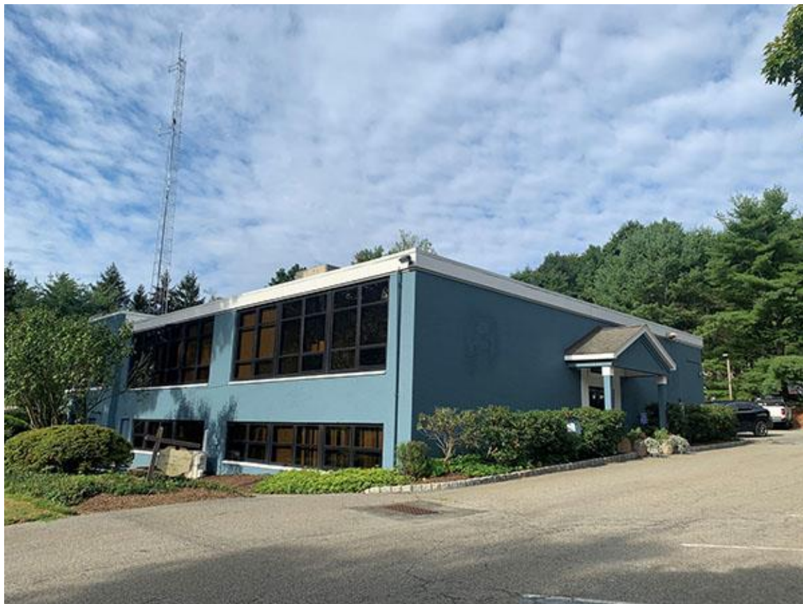
1952 Addition: Glass at Dais Area, Communications Tower
