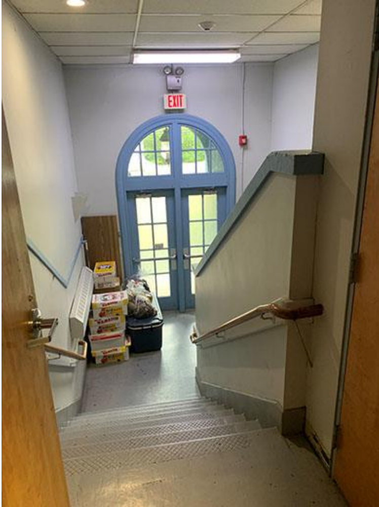
Existing Original Stair: Storage Challenges, Temporary Egress Issues
