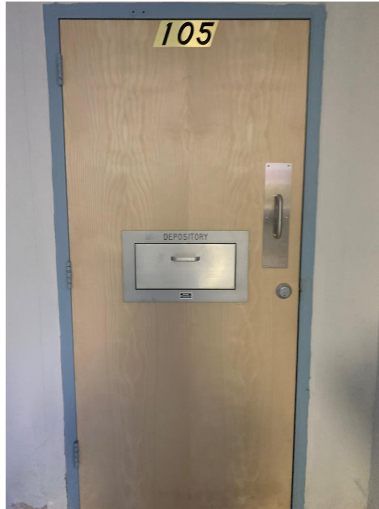
Evidence Storage: HVAC System Deficiencies, Security Controls
